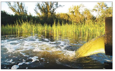
Outflows reached maximum discharge from Jordan Marsh approximately 24 hours after the large rain events of September 12 and 13, 2020. On September 14, the discharge reached 2,000 gallons per minute (normal discharge rate is under 1,000 gallons per minute).
